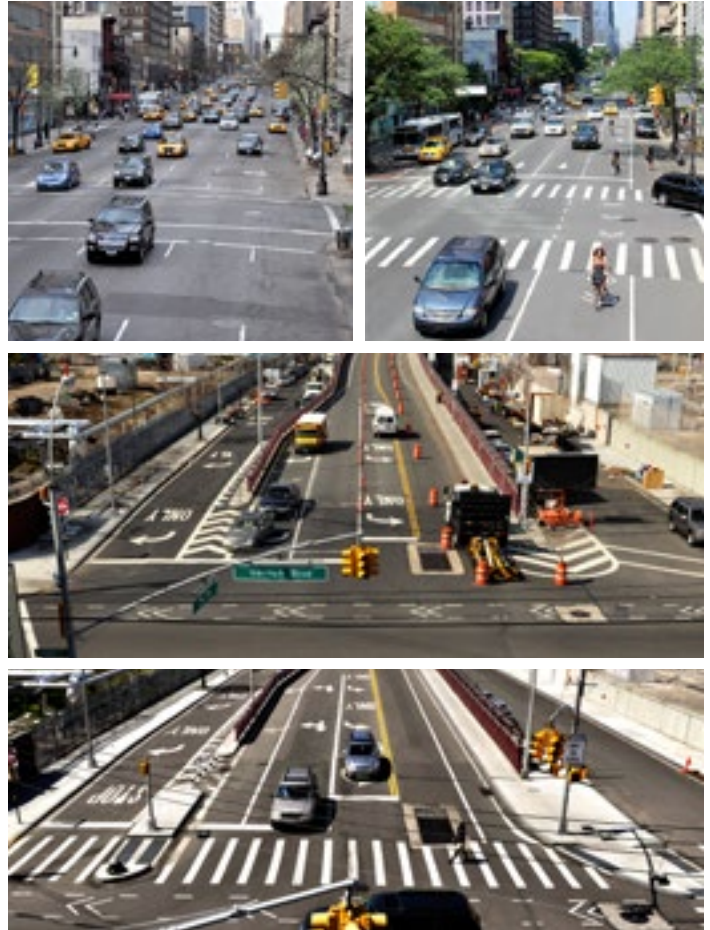
Complete streets, such as these retrofit projects in New York City, create a safe and welcoming environment for different types of road users including pedestrians, cyclists, cars, and transit vehicles.
