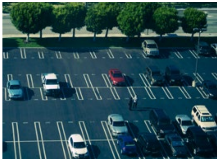
Parking facilities, such as this garage in Sunnyvale, California, and surface lot in Long Beach, California, are currently a dominant feature of American cities, suburbs, and small towns. Reduced parking needs as a result of AVs will provide opportunities to rethink and redevelop these areas.
