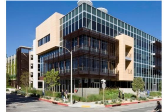
New medical research facility to support Palmdale Regional Medical Center.
