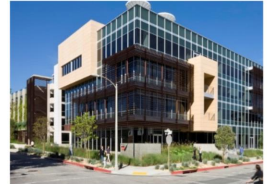
New medical research facility to support Palmdale Regional Medical Center.
