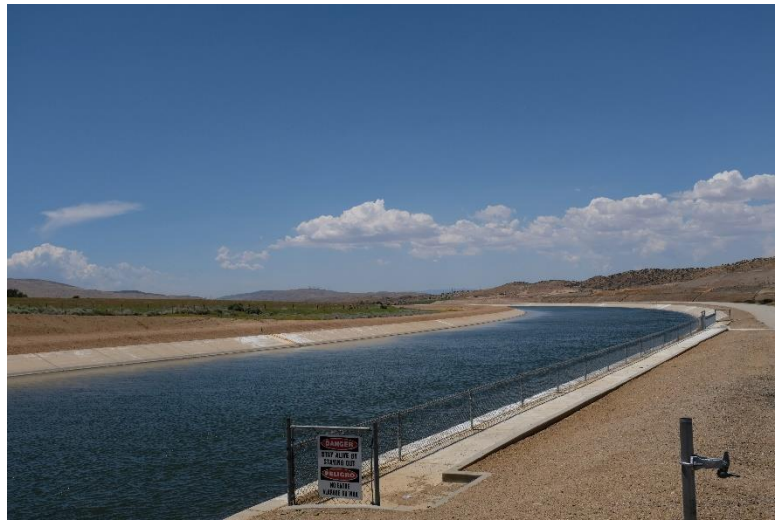
California Aqueduct in Palmdale.
