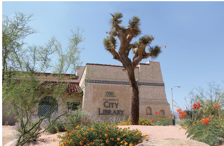
City of Palmdale Library
